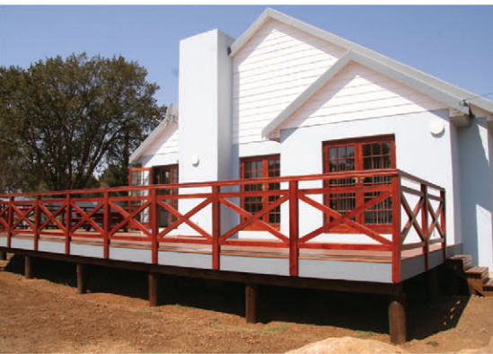
New build - Timber frame home
